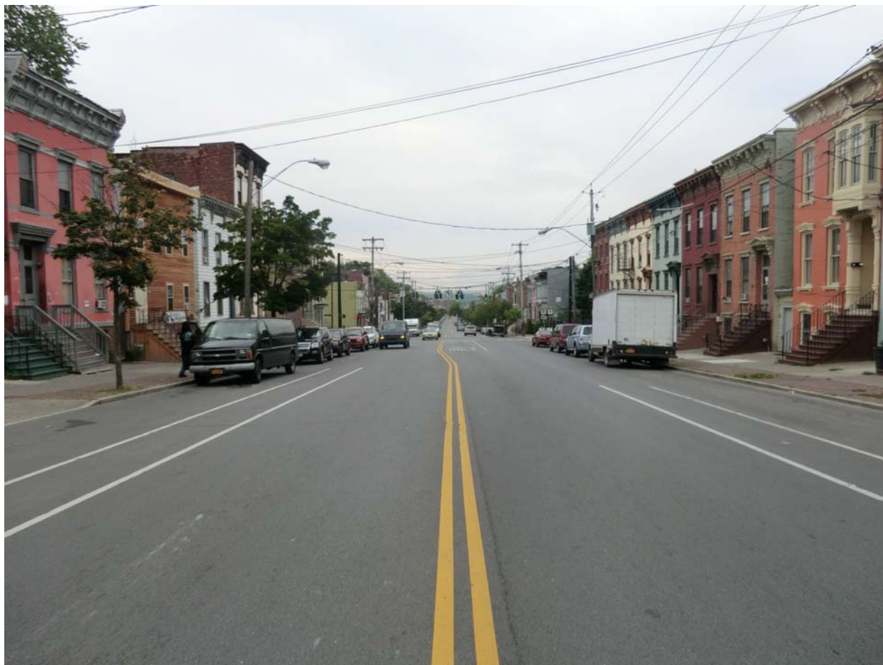
Clinton Avenue Bike Lanes and Intersection Turn Lane
