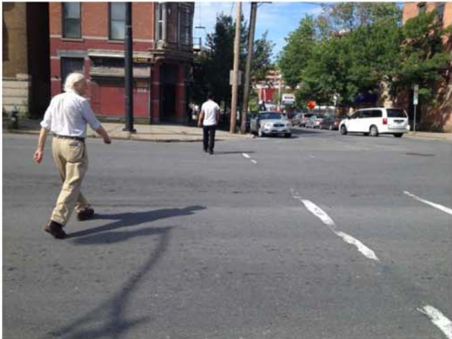
Worn crosswalks at Madison Ave and Knox St
