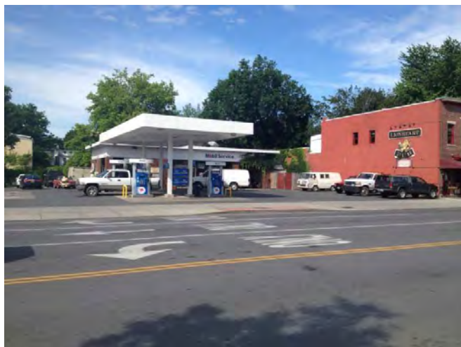
Mobil Station at Lark St and Madison Ave with wide driveways
